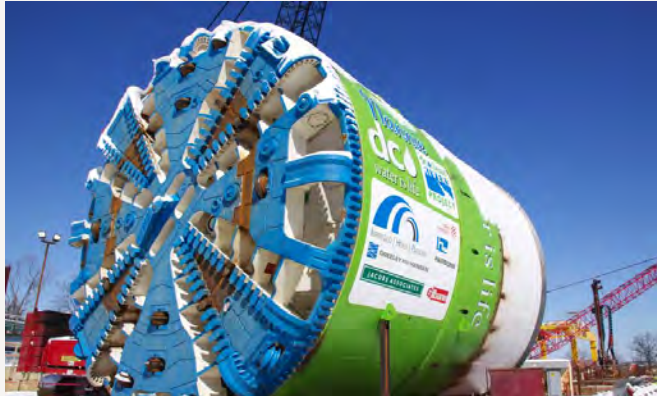
DC Water / Clean Rivers Program: 15 miles of 23 ft. diam. sewers - $2.6B
