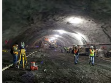
NYC Transit / Second Ave. Subway: 2 miles, 22 diam. transit tunnel - $4.5B
