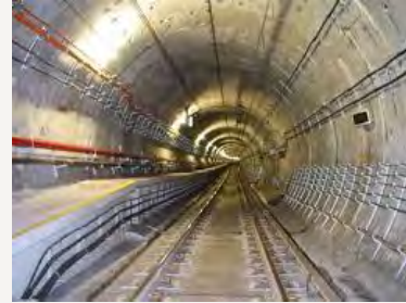
Northeast OH Regional Sewer District / Euclid Creek Tunnel: 3.4 mi., 24 ft. diam. ww tunnel - $199M
