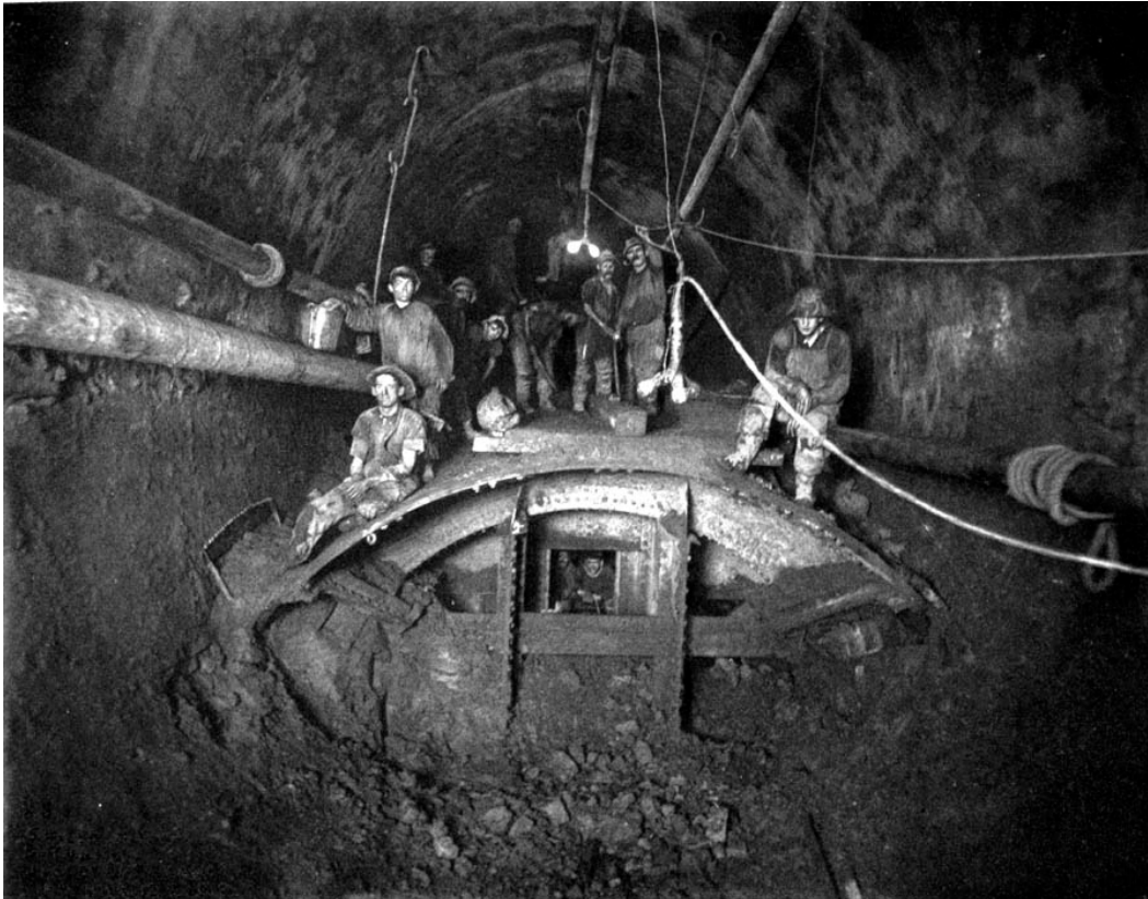
Figure 8 – Mechanical mole (TBM) of 1909 vintage, used to excavate the Hudson River Railroad Tunnels (now PATH) connecting lower Manhattan with New Jersey. (Archival image.)
