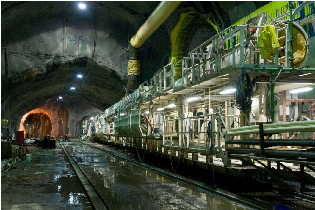
Figure 2 – View N within excavation for the Jacob Javits Convention Center station cavern of the MTA’s #7 Line Extension. To the right note that the hard-rock TBM and trailing gear has begun tunneling. (Web image.)
