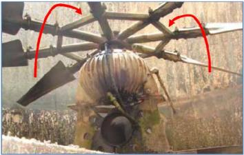
Figure 15: Fan Assembly- The fan assembly in the west cell is missing the FRP disk seal. The red arrows display the vacuum that is created at the fan hub causing air to re-circulate the fan assembly.
