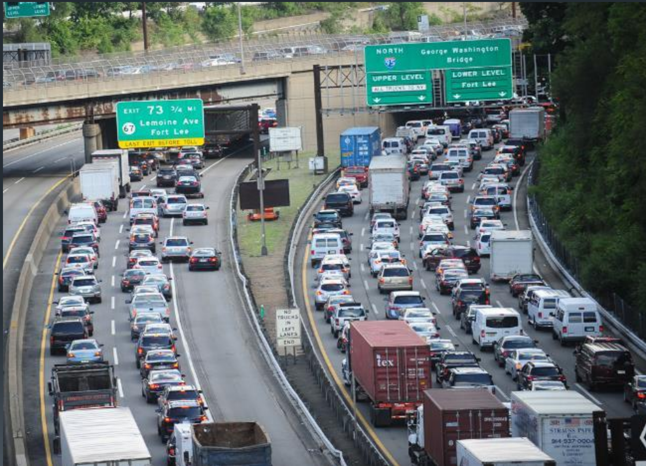
George Washington Bridge approach Fort Lee, NJ
