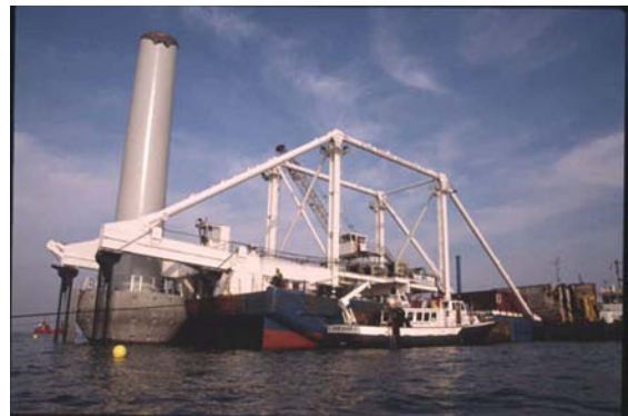
Figure 14: The floating crane with a foundation and the lower part of the tower at the site just before placing
