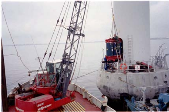
Figure 10: Transformer passing the door in the tower.
