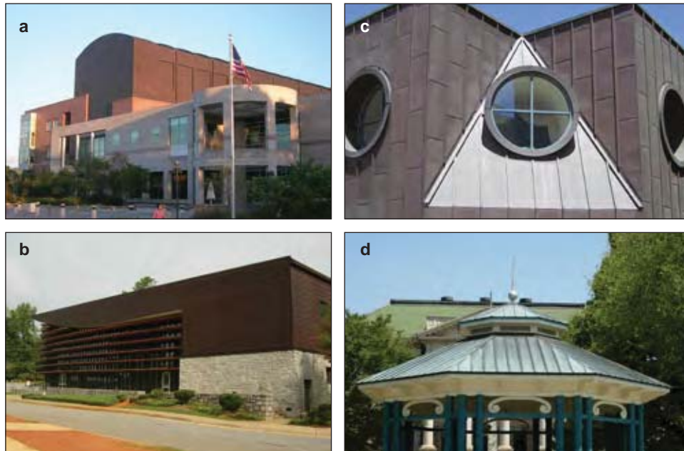
Figure III-8. The two figures on the left show typical weathering on vertical surfaces, while those on the right show how weathering differs on sloped surfaces. a) Sam Noble Museum, Norman, Oklahoma, semi-arid climate, 12 years after installation; Solomon+Bauer+Giambastiani Architects and Kaighn Associates Architects; b) Georgia Public Health Lab, Atlanta, Georgia, humid climate, 12 years after installation, Lord Aeck & Sargent, architect. c) Denver Public Library, Denver, Colorado, semi-arid climate, 17 years after installation, Michael Graves, architect; d) Gazebo, Decatur, Georgia, humid climate, 15 years after installation, Edwin Terrel Meek / Architect.
