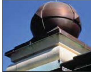
Figure IV-10. Copper globes, fabricated from spun and brake-formed components, adorn four towers at the corners of the Ellis Island Immigration Museum in New York Harbor, New York, New York.
