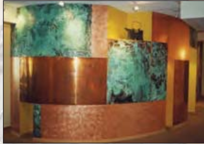
Figure VI-1. This lobby in Anchorage, Alaska, artfully displays panels of copper alloys using a variety of colorful chemical and mechanical finishes.
