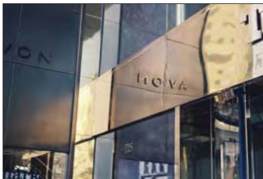
Figure VI-3. The specular or mirror finish on this facade reflects the colors and images of its environment.
