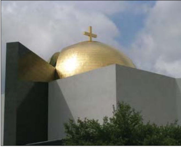
Figure VI-13. Gilded copper dome crowns the Chapel of St. Basil in Houston, Texas; Niko Contracting, sheet metal installer.
