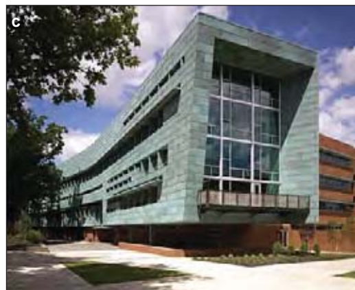
Figure I-4. a) Heat-treated and chemically weathered panels at the National Museum of the American Indian, Washington, D.C. b) Ornate flashing, finials and cresting on New York's Engine Company 31, naturally weathering since 1896, New York, New York. c) Prepatinated copper facade on Penn State's School of Architecture and Landscape Architecture, State College, Pennsylvania.
