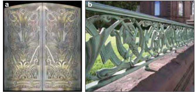
Figure IV-6. a) These art deco sliding doors are cast from C83700 silicon bronze and are modeled after antique elevator doors found at the Essex House Hotel in New York City. The visible surface is sand-cast bronze. Highlights were polished and brushed before application of clear lacquer coat. b) This beautiful bronze railing in San Francisco, California demonstrates long-term weathering tones characteristic to many areas.
