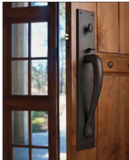
Figure VI-7. The oxidized finish on this cast silicon bronze lockset produces a stable compound that inhibits corrosion and maintains its color.
