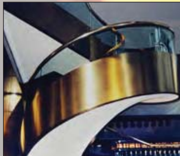
Figure IV-2. Copper alloys installed on this staircase at the European American Bank, New York, New York are examples of simple bending. The handrail is a solid extrusion of architectural bronze, C38500; stringer cladding is Muntz metal, C28000.
