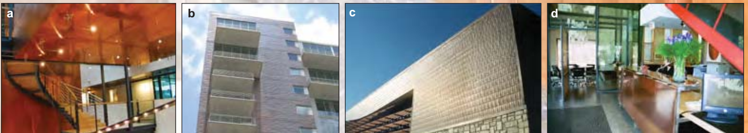
Figure V-1 a) Flat, mirror-finish copper clads the interior of the Finnish Embassy; Washington, D.C. b) The oil-canning typical in light gauge sheet metal adds texture to the face of the City Lofts building in Austin, Texas; Pageg Southerland Page, Architect. c) Striking wall cladding of stamped copper shingles distinguish this Atlanta, Georgia lab building; Lord Aeck Sargent, Architect. d) A polished copper panel and countertop highlight this reception area.
