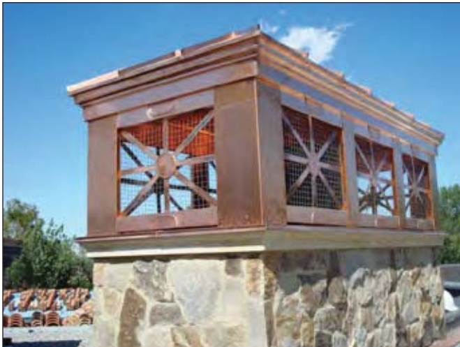
Figure IV-15. Seamed and mechanical joints were employed to fabricate this chimney cap.
