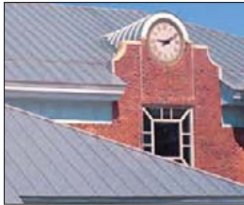
Figure II-3. The pleasing, naturally weathered, soft gray color on this roof and dormer is provided by lead-free, tin-zinc coated copper from Revere Copper Products.
