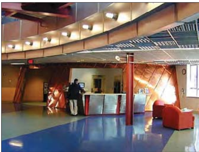
Figure IV-13. Seams between individual sheet copper panels create a decorative pattern in the vestibule of Central Connecticut State University's Student Center in New Britain, Connecticut.
