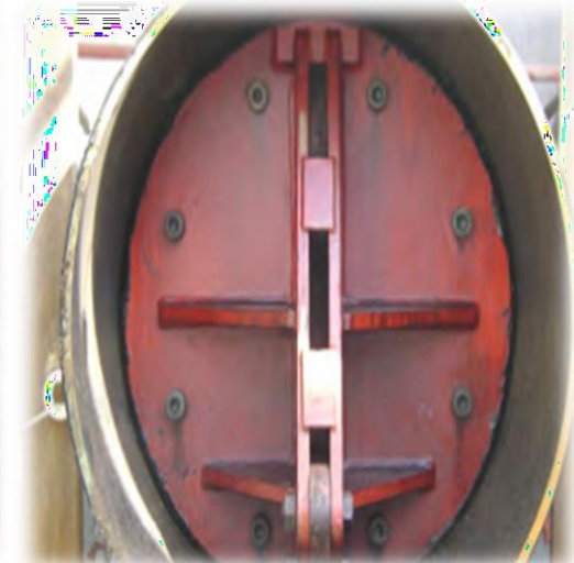
LINE STOP PLUGGING
