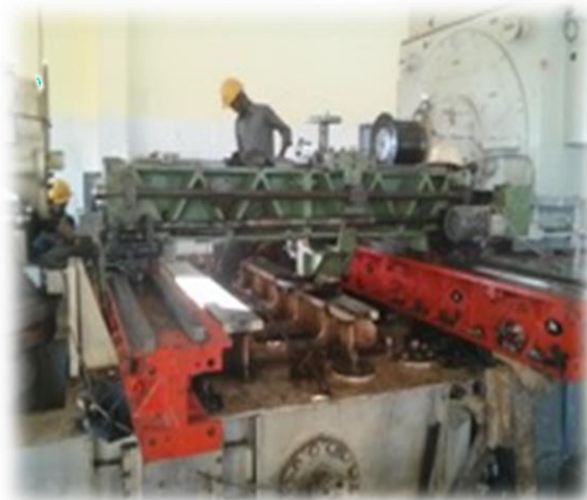
In-situ Milling – Gear box seat
