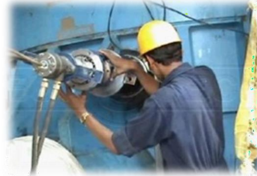
Gear Box Dowel Hole Machining
