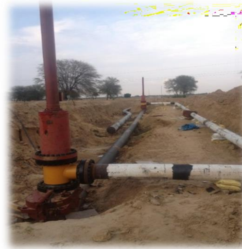
LINE STOPPLING PROCESS
