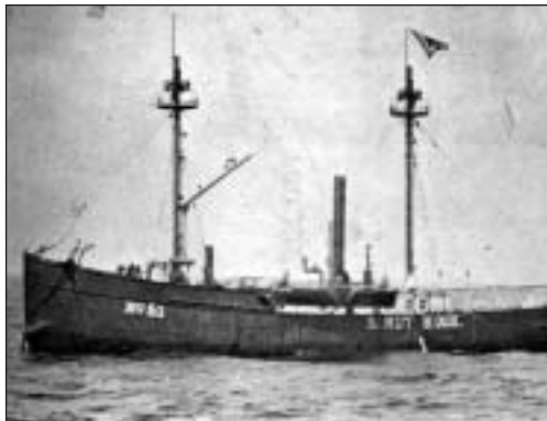
LV-51 served the Sandy Hook station from 1894-1908.
