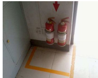
Example of area in front of fire equipment kept clear.
