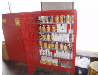
Proper storage of flammable liquids in a designated and properly designed cabinet.
