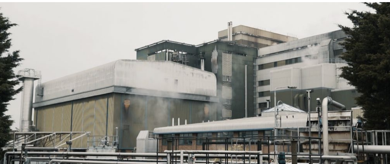
JDE Banbury, United Kingdom Manufacturing Facility
