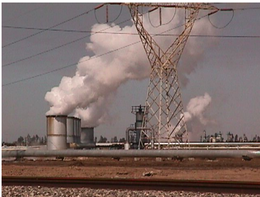
Figure 16. A humid corrosive environment in a geothermal field caused by steam and gases emission.
