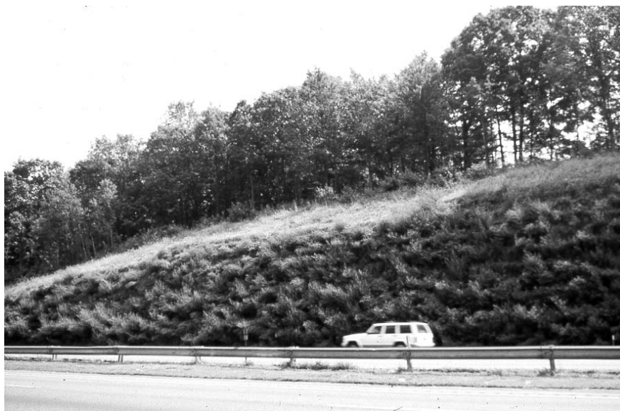
Figure 8-11. Massachusetts Turnpike during construction, immediately after construction and the after the second growing season.
