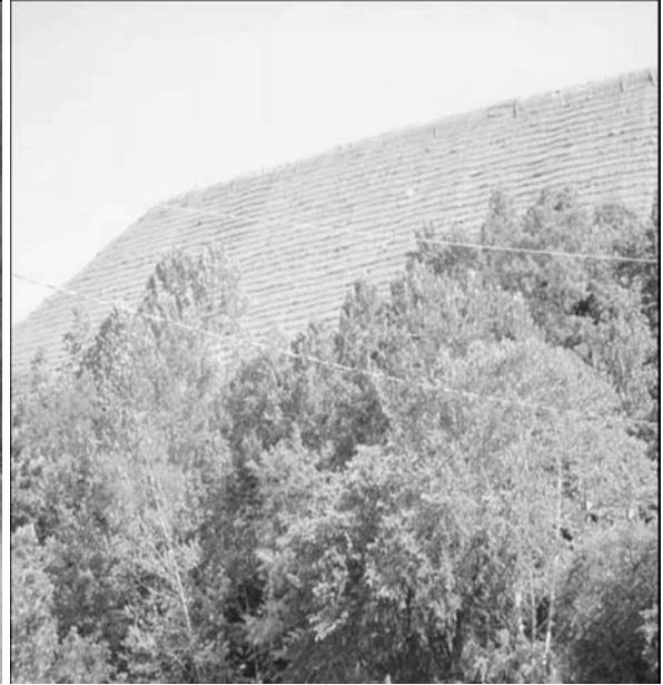
b) Slope face during construction.
