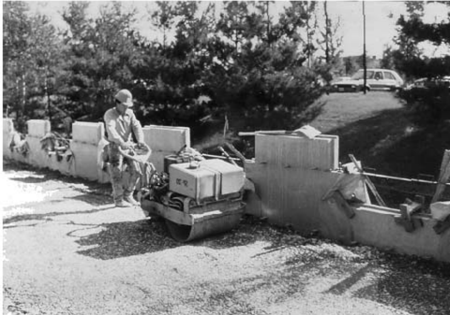
Figure 11-8. Compaction equipment showing: a) large equipment permitted away from face; and b) lightweight equipment within 3 ft (1 m) of the face.
