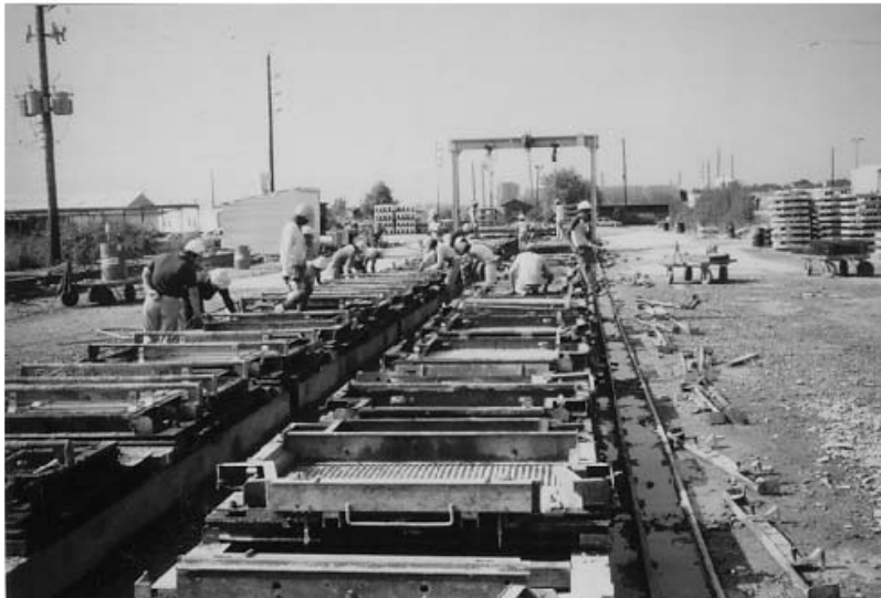
Figure 11-1. Casting yard for precast facing elements.
