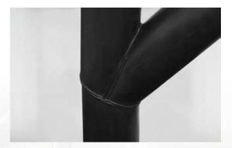
In this technique, both pipe ends are pressed against a hot plate at a constant temperature and pressure. Then pipe ends are pressed on head to head situation so that both pipe ends are fused together.
