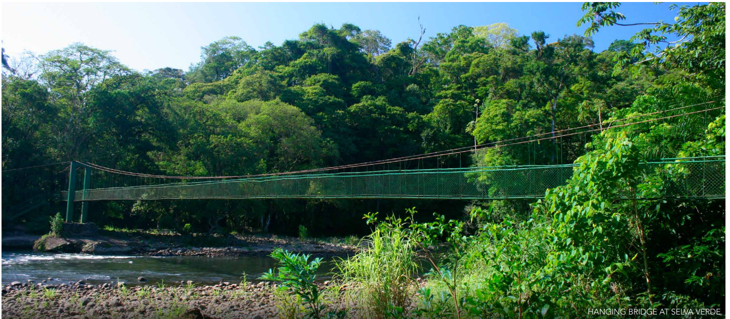
HANGING BRIDGE AT SELVA VERDE
