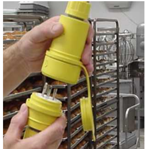
Figure 5- Unplug equipment prior to cleaning
