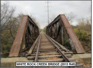
WHITE ROCK CREEK BRIDGE (2013 R45)
