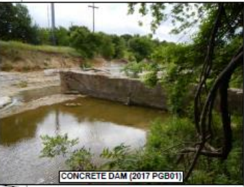
CONCRETE DAM (2017 PGB01)
