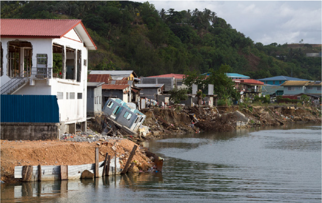
// Image 3. Damaged buildings along Mataniko river, Honiara, post-2014 floods ©UN-Habitat
