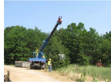
Transformer relocation
