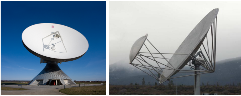
Figure 15: A Cassegrain antenna (left) Gregorian antenna (right)
