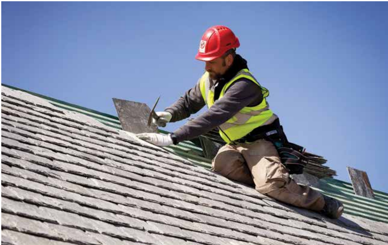
Trevillet Slate being laid at Tregunnel Hill
