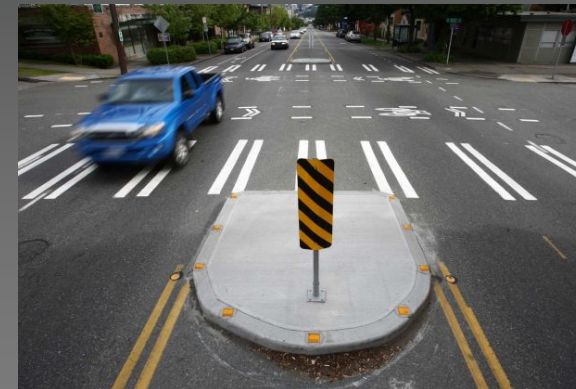
Figure 17. Shared lane marking
