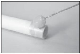
Apply a heavy, even coat of cement to the outside of the pipe end. Work the cement into the joining surfaces using a continuous, circular motion.
