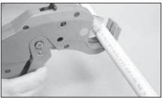
Be careful not to split the pipe if using a ratchet-type cutter, especially in temperatures below 50° F. If any damage or cracking is evident, cut off at least 2" of the pipe beyond any visible crack.
