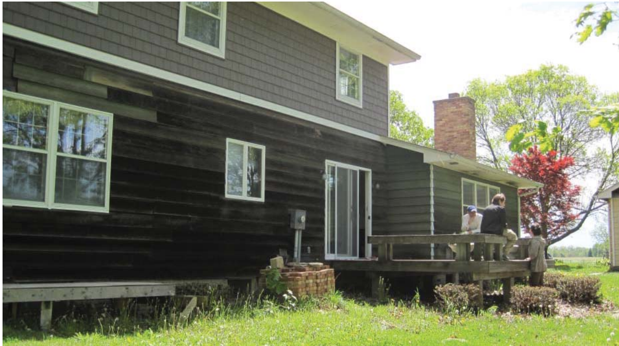
Existing north facade of Schmedeke residence
