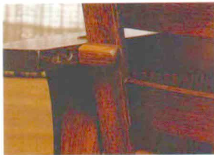
Back adjustment pegs (above) fit into holes in the arms. Moving the peg back allows the chair back to recline.
