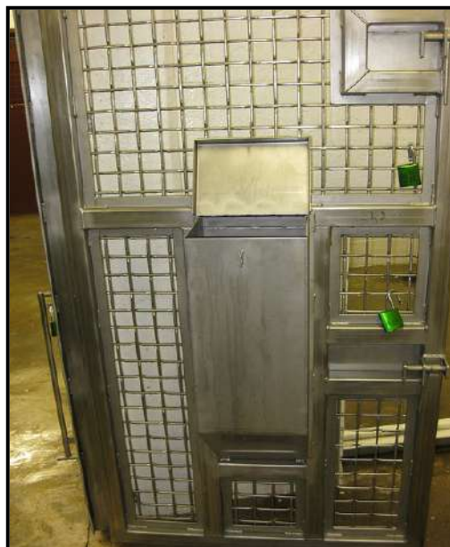
Food chute, keeper side. M. Waagner
