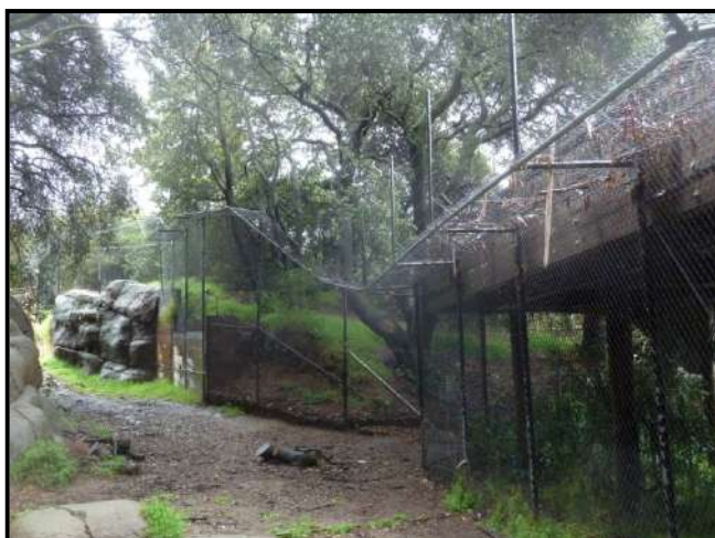
Chain link fence barrier with 90 degree turnback M. Jeffries
