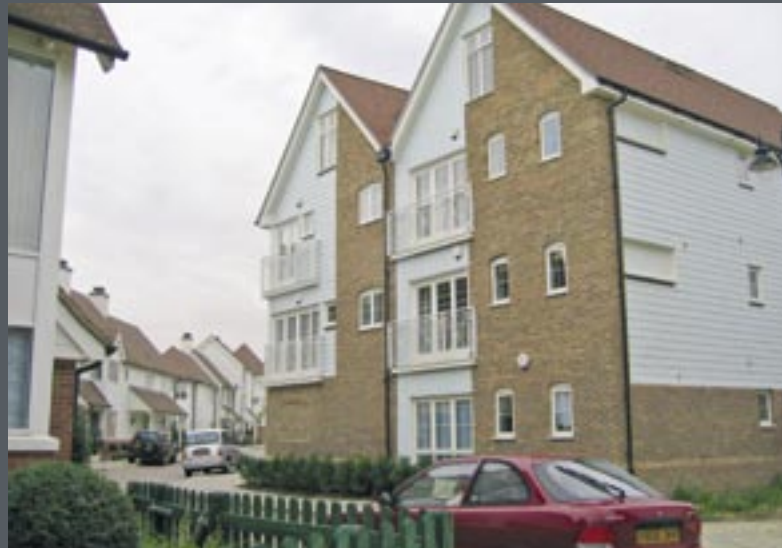
7 Buildings that provide a sense of enclosure to the street.
