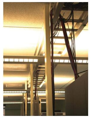
Illustration 4: The "ladder" carrying network cabling between rows of workstations. Note the bundle of cables rising obliquely from the server rack (right foreground) to the ladder, and vertical bundles of cables running from the ladder down to the trough below (not shown).
