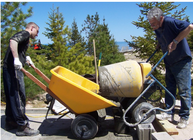
Jeremiah Hartwell and Rick Brockway mixing concrete.
