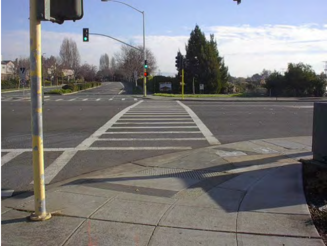
FIGURE V-7. Looking east from southwest corner of Atlantic/Constitution intersection (Section 2).
