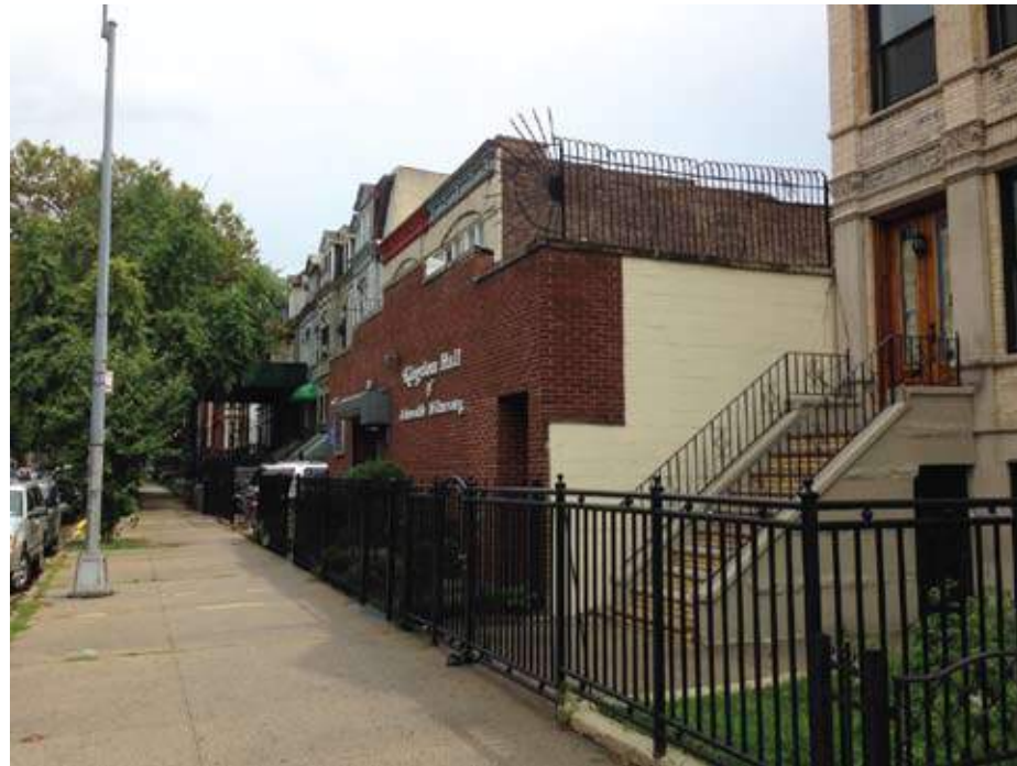
3 VIEW OF EXISTING FACADE LOOKING WEST
