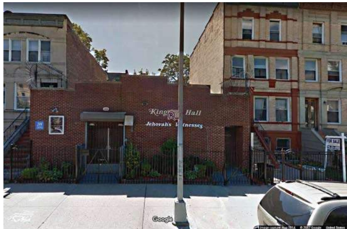
3 EXISTING FRONT (SOUTH) PHOTO
