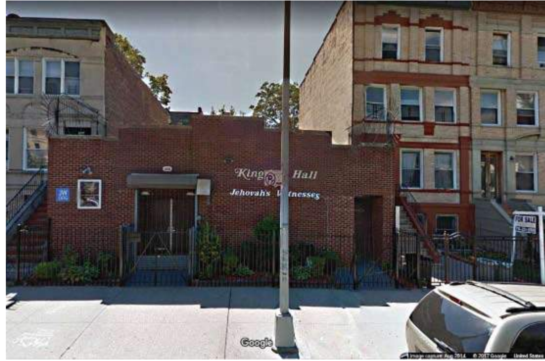
2 VIEW FROM ACROSS THE STREET OF EXISTING FACADE (SOUTH)
