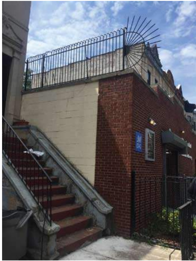
1 VIEW OF EXISTING FACADE LOOKING EAST
