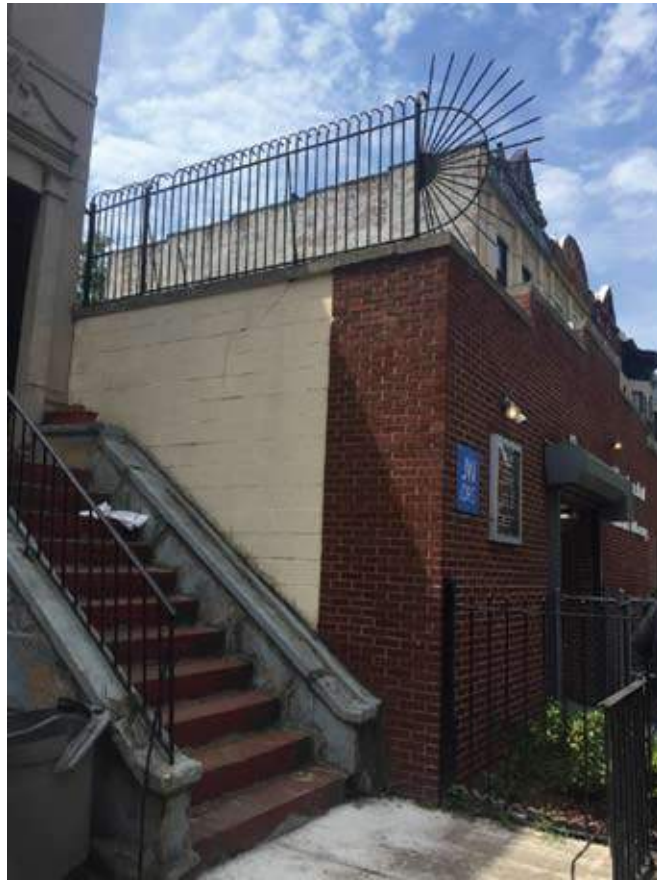
1 VIEW OF EXISTING FACADE LOOKING EAST
