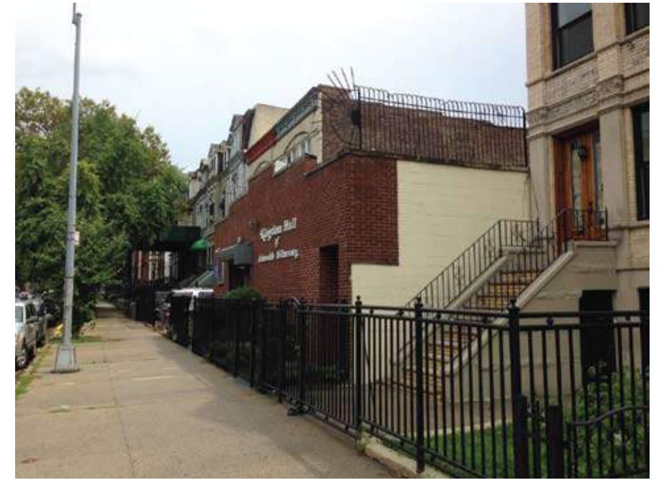
3 VIEW OF EXISTING FACADE LOOKING WEST
