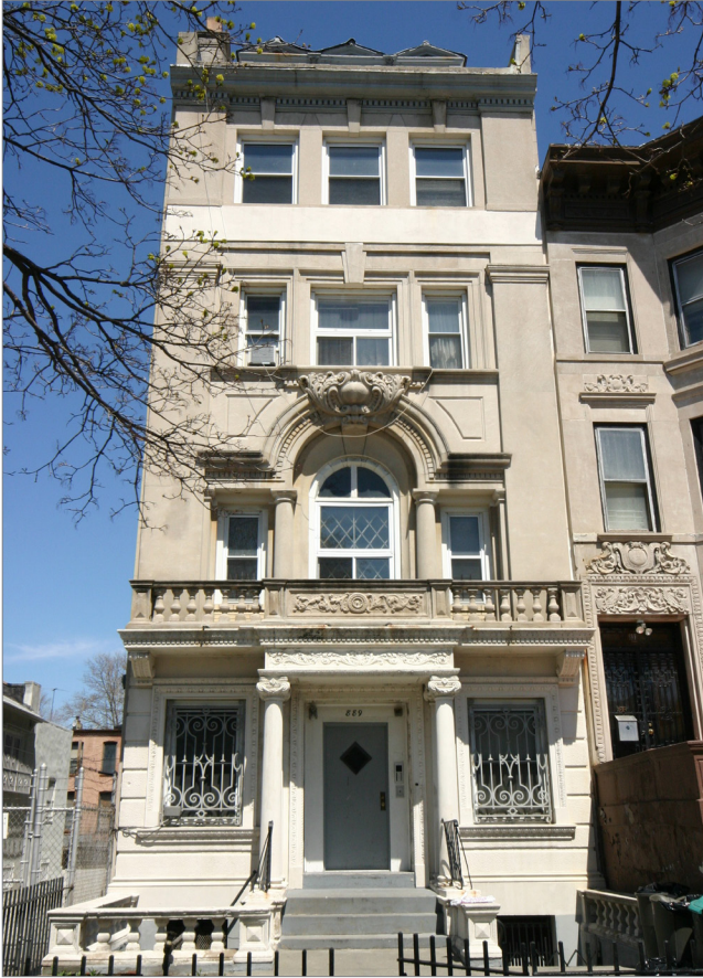
889 St. Marks Avenue. Image courtesy of the Landmarks Preservation Commission
