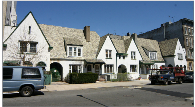
935-947 Prospect Place. Image courtesy of the Landmarks Preservation Commission
