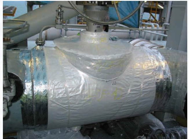
Cryogenic valves before and after being insulated with Cryogel® Z.
