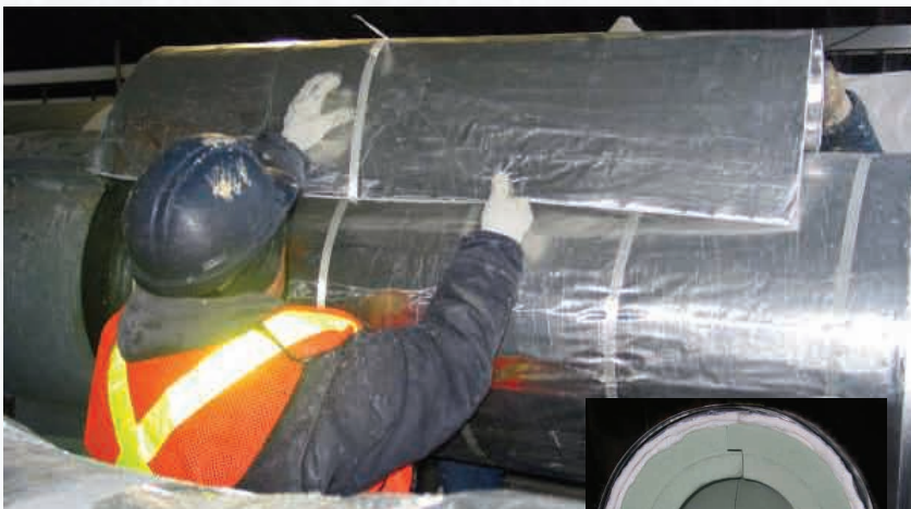
Contractor installing two layers of Cryogel® Z over PIR pipe cover.
