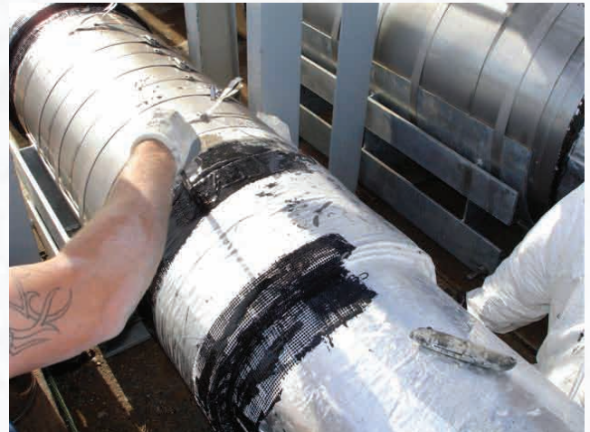
Cryogel® Z tie-in to adjacent insulation material.
