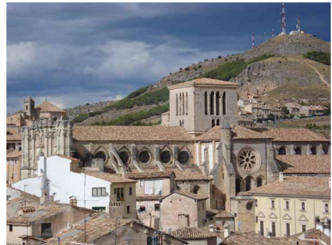
Fig. 2.15 Cuenca Cathedral, view from the southwest (2007).
