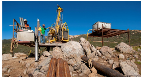
Figure 3: Crews Complete Micropile Installation on Sunrise
