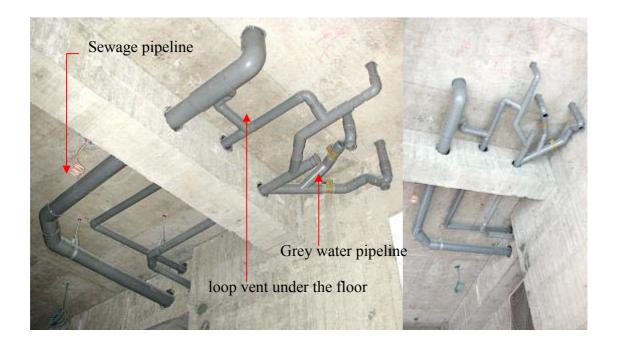
Figure 11 Picture of partial drainage piping work under floor
