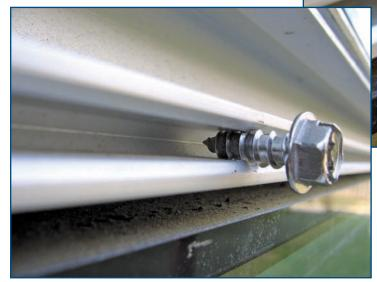
nections could be easily stripped due to the relatively shallow engagement of the pressure-plate screws and the somewhat oversized screw chase (*Figure 6*). Corrosion of the aluminum screw chase was noted at nearly all of the upper screw sites at the sunshade with the pressure-plate screw connection failure. Many stainless-steel pressure-plate screw sites exhibited similar corrosion; *Figure 7* illustrates a location with relatively severe corrosion.
