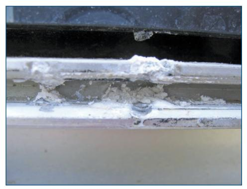
Figure 7 – Severe corrosion of aluminum screw chase.
