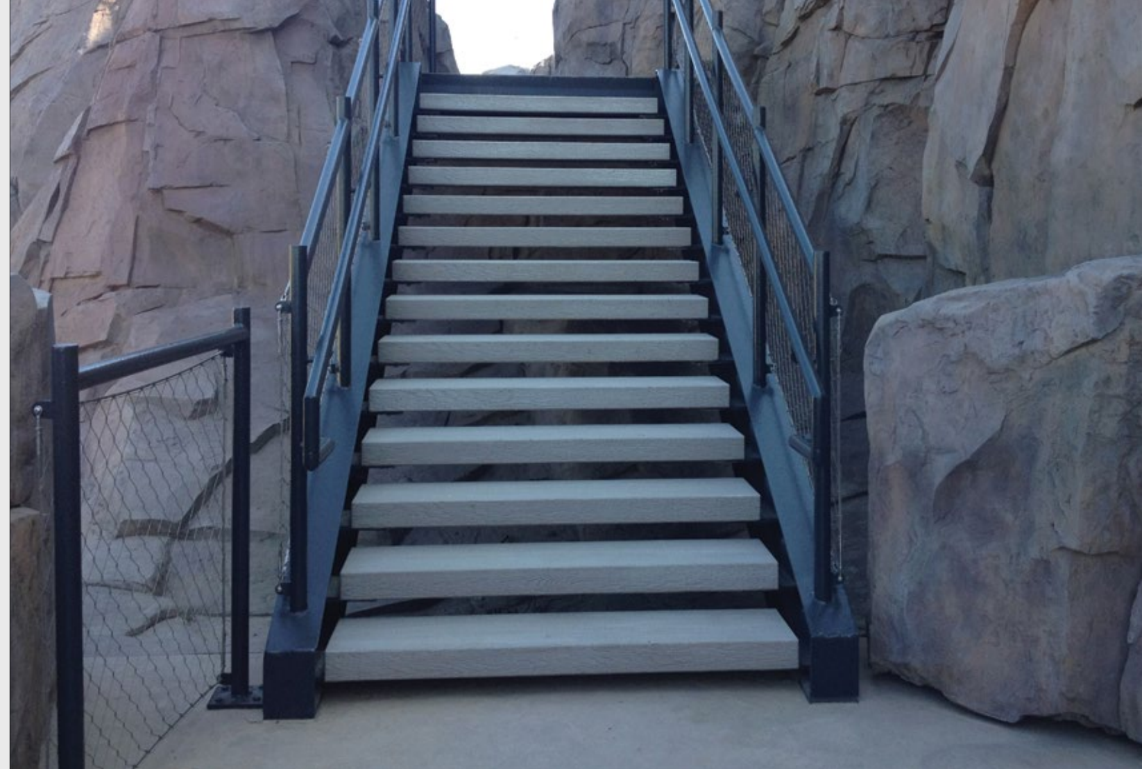
Epic Headquarters | Verona, WI | Custom Precast Concrete Self-Supporting Treads
