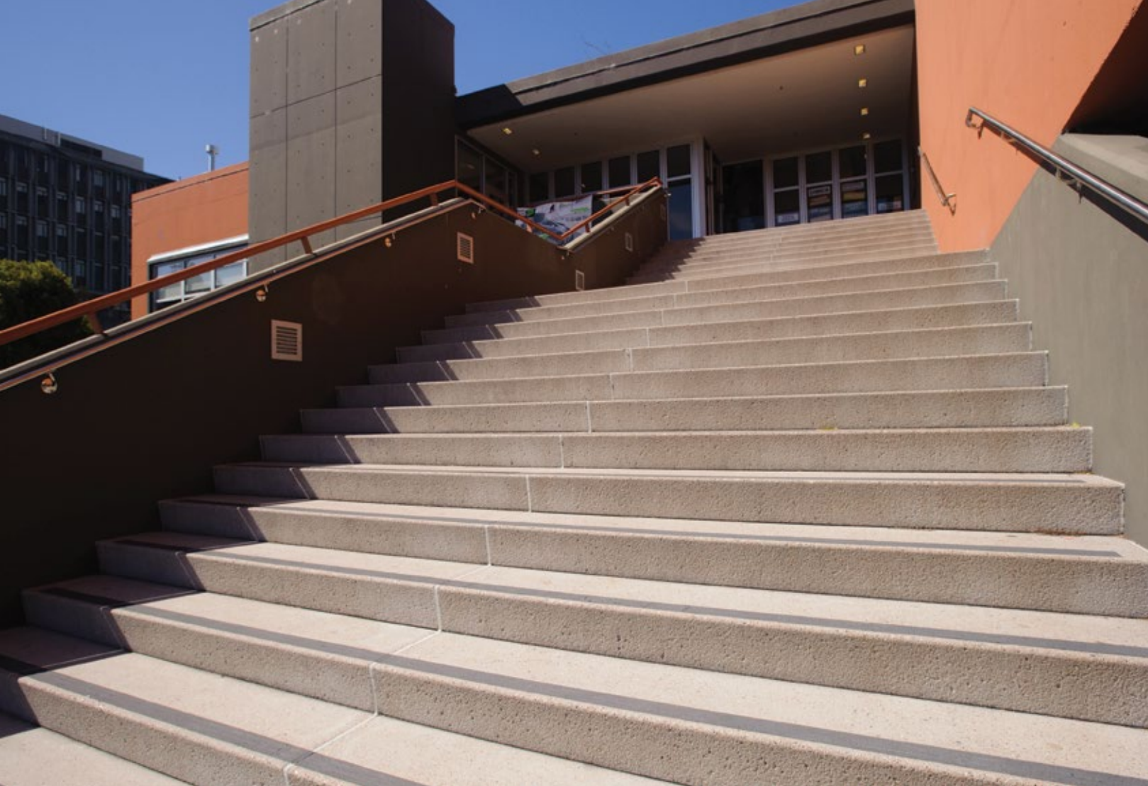
Harvey Milk Photo Center | San Francisco, CA | Custom Precast Concrete Fully-Supported Tread and Risers
