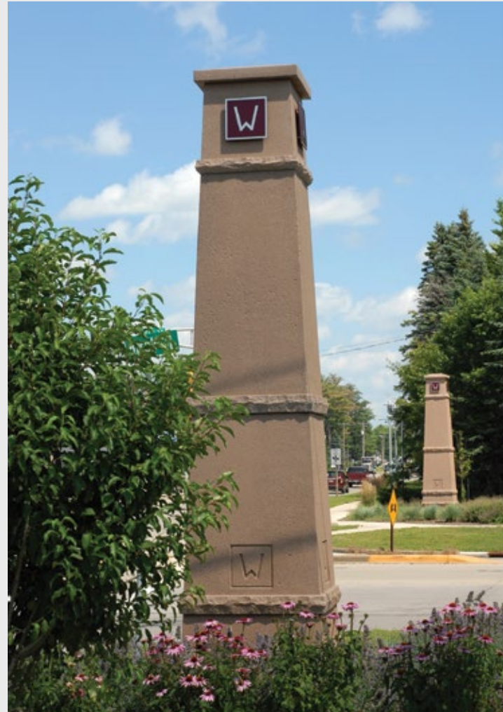
Schofield Ave. | Weston, WI | Custom Precast Concrete Columns
