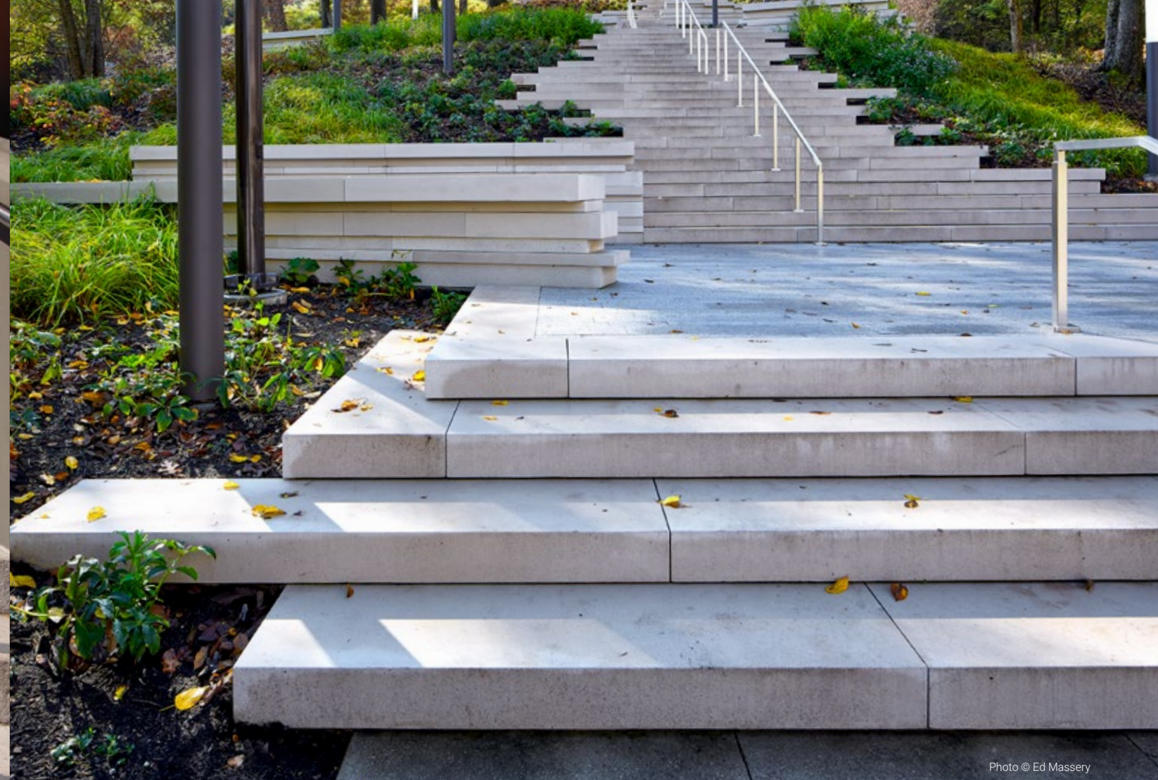
Art Climb | Cincinnati, OH | Custom Precast Concrete Fully-Supported Tread and Risers
