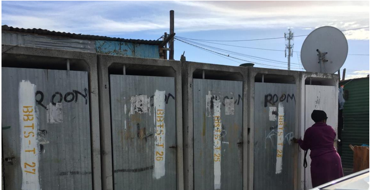
Figure 13 Shared toilet facility in Khwezi Park 45
