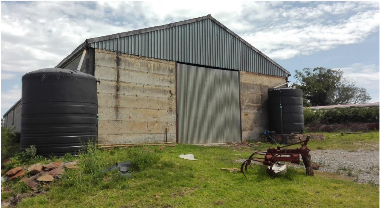
Figure 19 Water storage tanks at business premises 48
