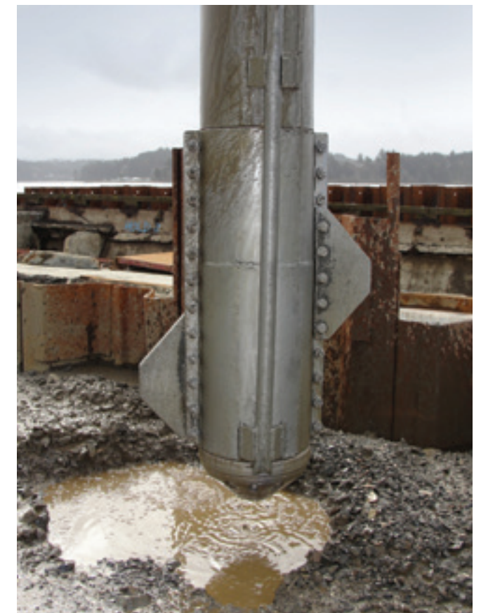
BELOW: Vibrocompaction, Port of Newport, OR
