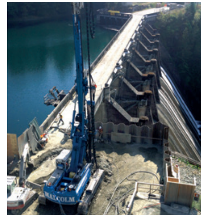
BELOW: Mega Jet Grouting, Ruskin Dam, British Columbia, Canada
