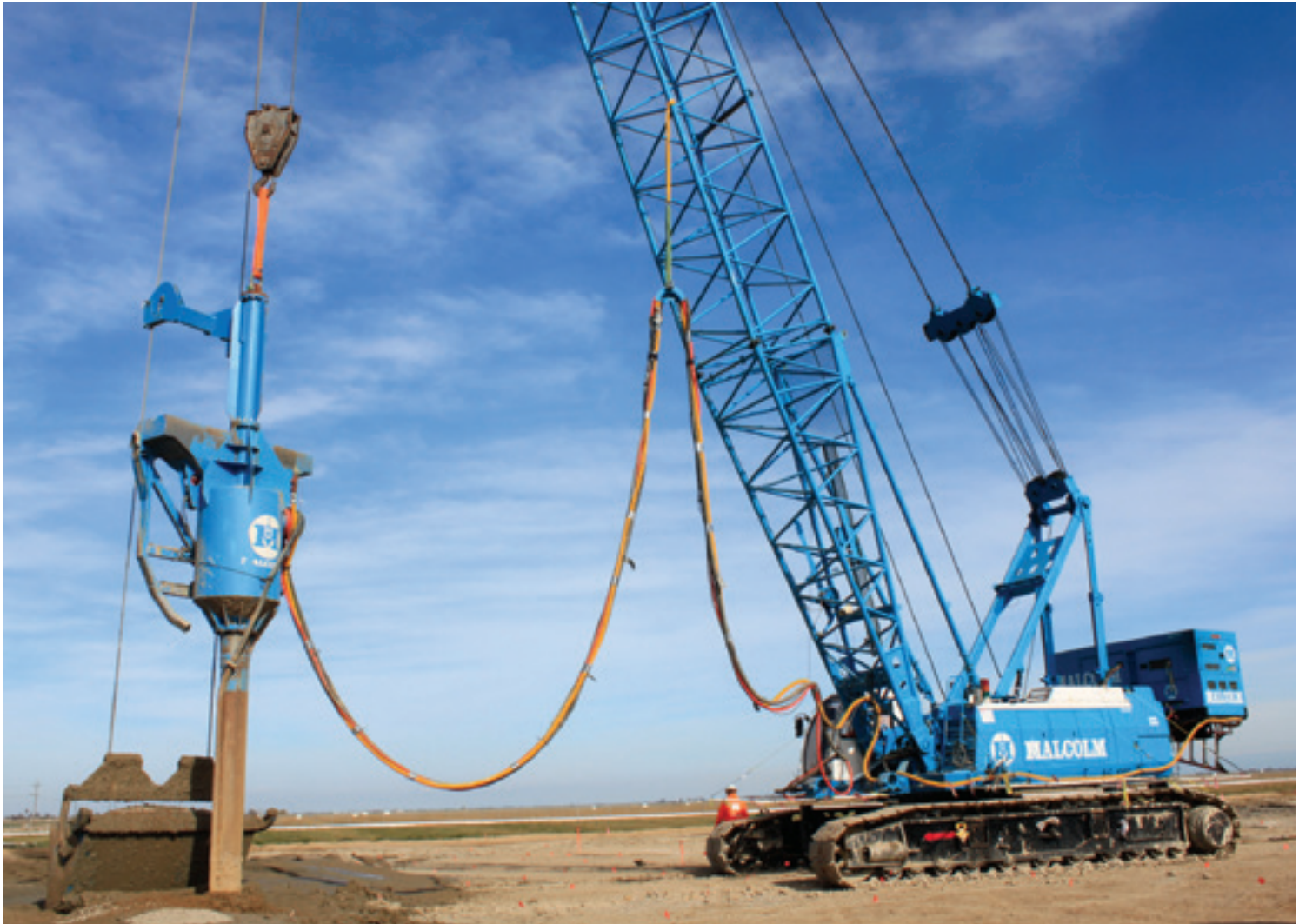
Front cover: Cutter Soil Mixing, Alaskan Way Viaduct Replacement, Seattle, WA
