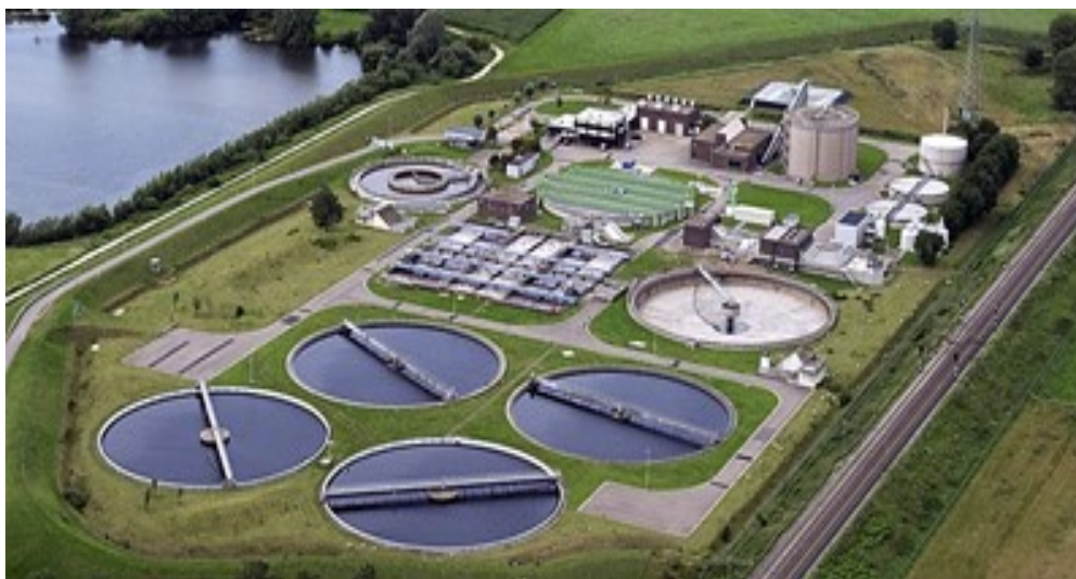
Figure 1.7: Sewage Treatment Plant[8]
