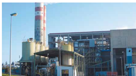
Waste Incineration Plant
