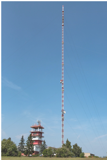
Fig. 5. The high power transmitter Brno - Kojál with antennas 305 m above the earth is effectively covering South and Central Moravia.
