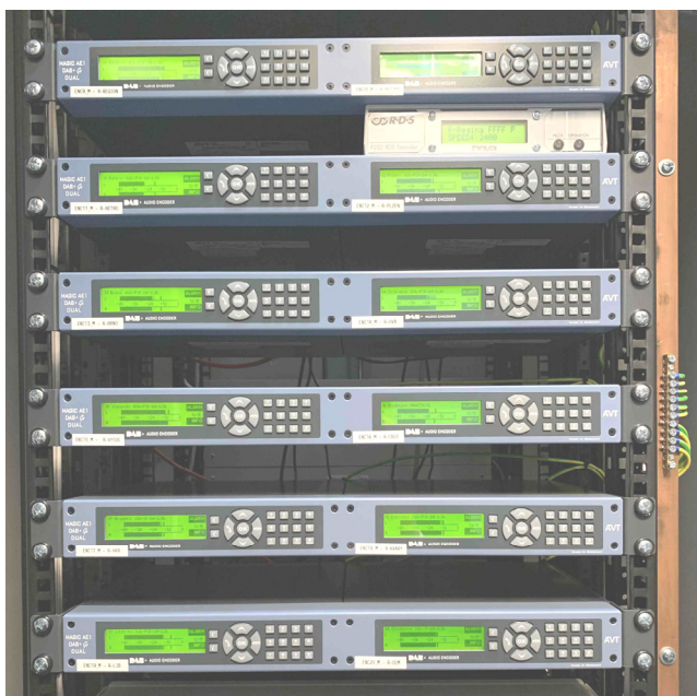
Fig. 10. The AAC audio encoders of the Czech Radio DAB+ network.
