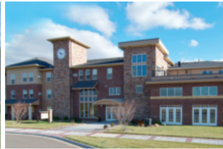
Vermillion River Crossing
