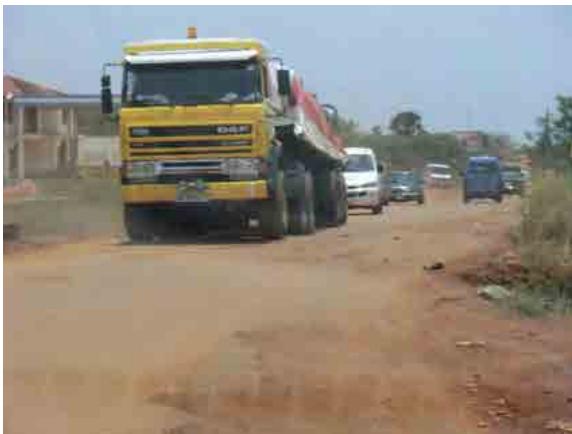
Unpaved section in Coastal Road Near the Togo borde, Ghana
