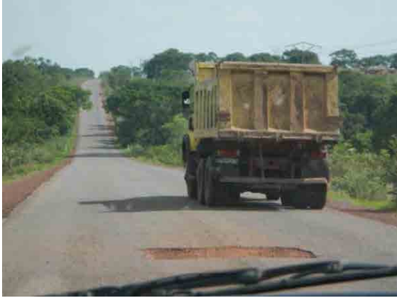
Road with pothole Bamfora-Niangoloko, Cote d'Ivoire
