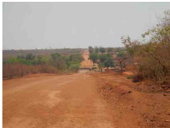
Section under rehabilitation Bella-Gaya, Niger
