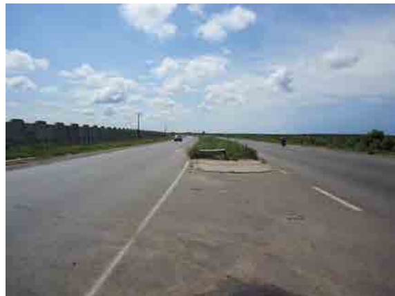
Paved section in Coastal Road Benin
