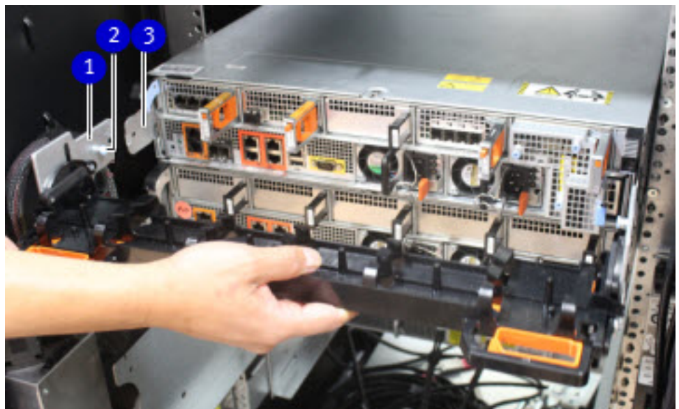
Figure 18 Installing the CMA
