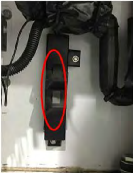
Figure 10.5 Supply Air Sensor Removal
