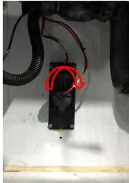
Figure 10.5 Supply Air Sensor Removal
