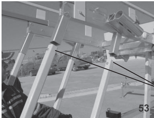
Figure 9 - Assemble Handrails
