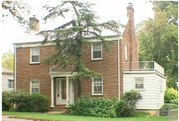
2001 Branch Avenue SE; 1939 District of Columbia Office of Planning; 2004
