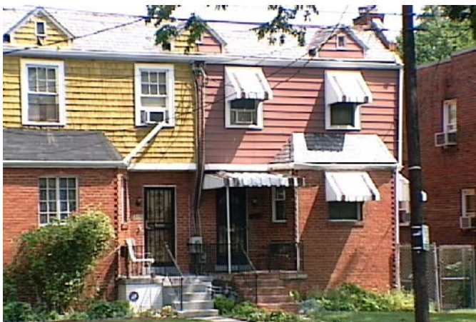
5312 East Capitol Street NE; 1935 District of Columbia Office of Planning; 2004
