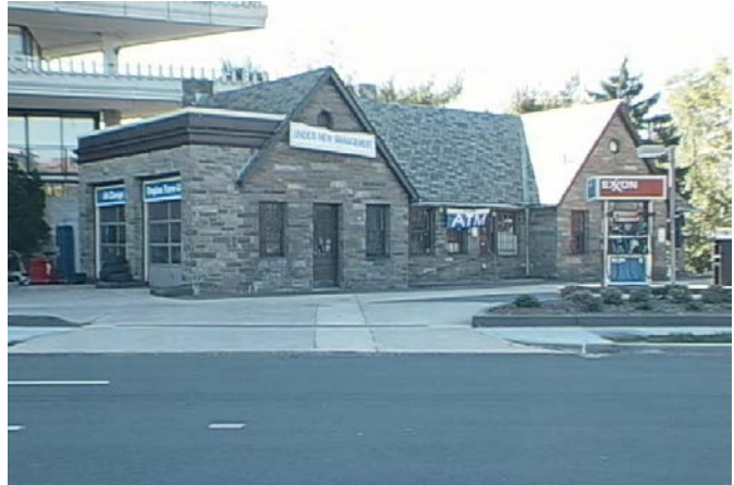
2708 Virginia Avenue NW; 1932 District of Columbia Office of Planning; 2004
