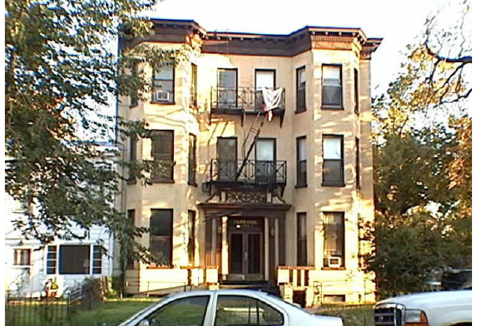
The Torraine, 424 East Capitol Street NE; 1905 District of Columbia Office of Planning; 2004
