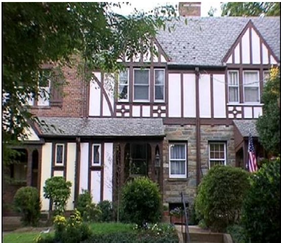
Tudor Revival Rowhouses, 4400 Block of Volta Place, Foxhall Village (1931)
