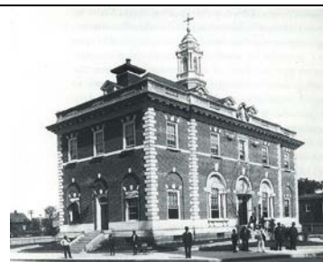
Post Office, Annapolis, Md. Lee, Architects to the Nation , 202
