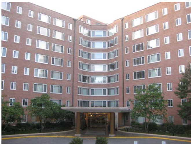
Quebec House Apartments, Connecticut Avenue and Quebec Street, NW EHT Traceries, Inc., 2010
