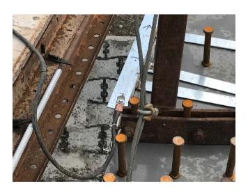
Support Angle with slot cut to facilitate hold down clip
