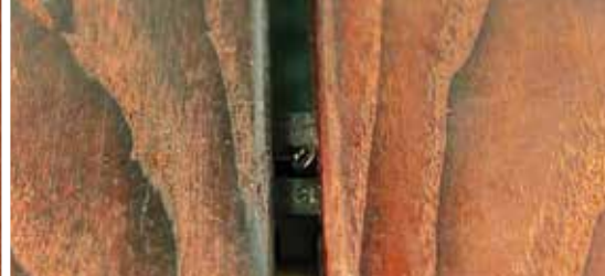
Hidden Deck Fastening Thermally Modified Woods
